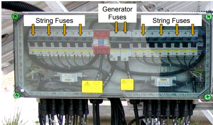
Fig. A6 - Array junction box
